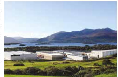
Liebherr container cranes in Killarney
