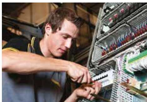
An electrical apprentice wires a cranes switch gear
