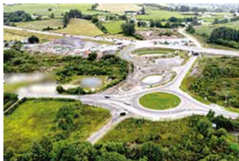
New road layout at the Macroom side of Ballyvourney, as the Macroom Ballyvourney Bypass nears completion. © Peter Scanlan
