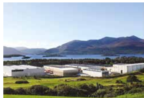
Liebherr container cranes in Killarney
