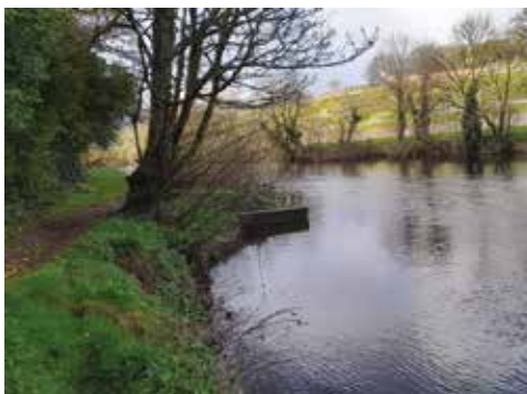
The outlet pipe behind Coleman's Park Treatment plant.
