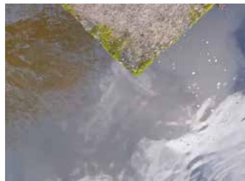
On the top of the concrete base of the pipe.
