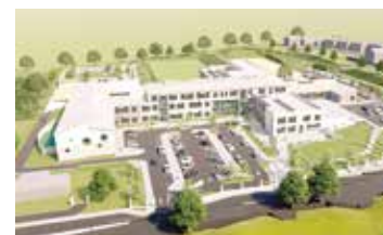
Coachford College. This new three story building will help the college to cater for over 1,000 pupils in the coming years.
