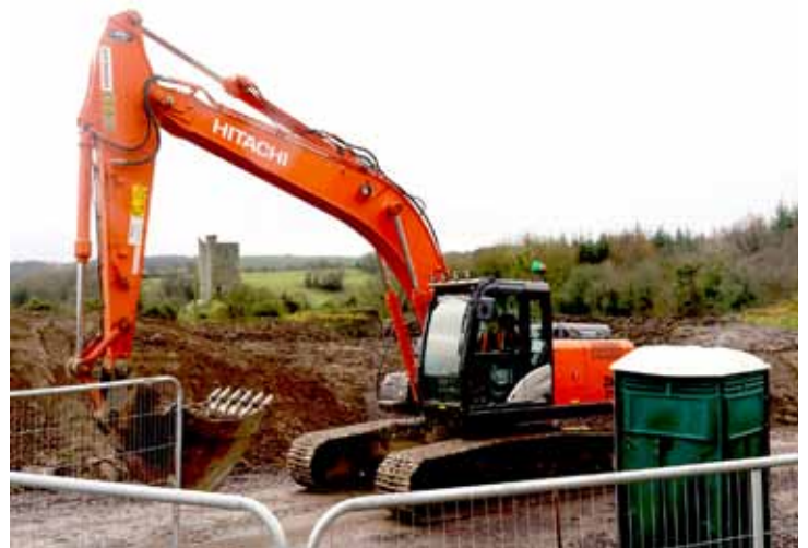
A modern digger frames old Carrigaphooka Castle at Carrigaphooka.(C. Kelleher).
