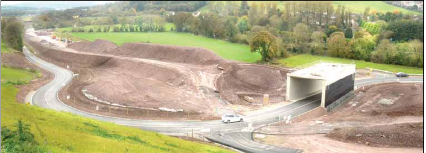
Progress on the Macroom Bypass © Peter Scanlan
