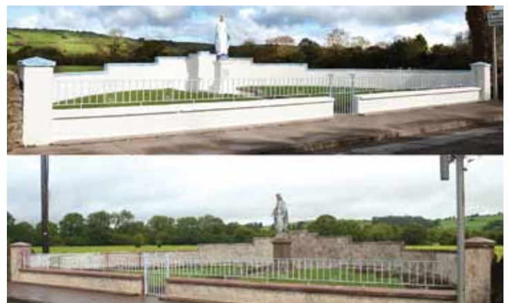
Marian Shrine Crookstown before and after refurbishment. © Peter Scanlan
