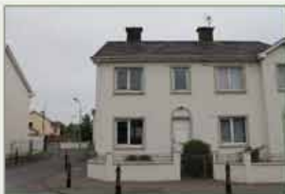
3 Na Tuir Cork Street, Macroom Co Cork. P12CV65.
