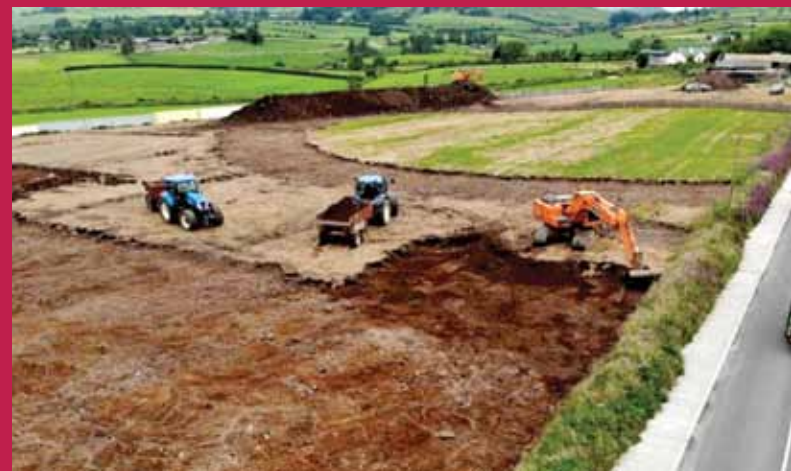
Work in progress for a new pitch in Rylane.
