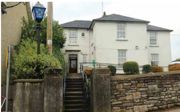
Macroom Garda Station, open and working. © Con Kelleher
