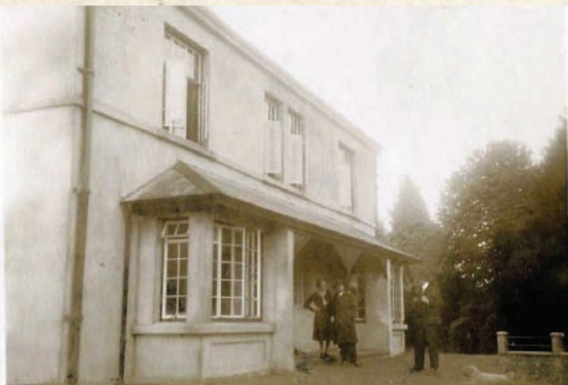
building just completed. 10th October 1931
