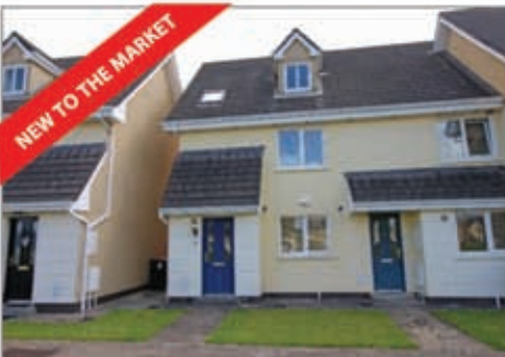
NO. 4 MANOR GREEN, GRANGE MANOR, OVENS, CO. CORK P31YR61
