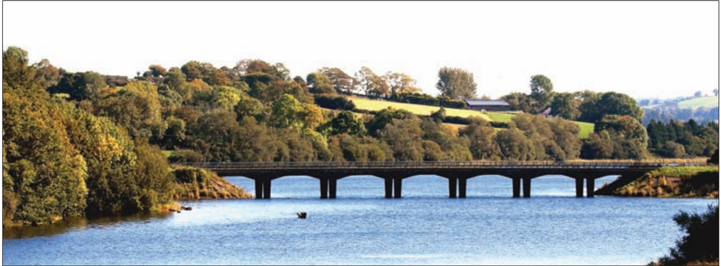
Coolcover Bridge in bright sunshine ©Con Kelleher
